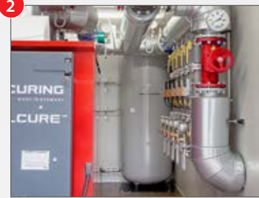
2 High-performance circulation pump available in bronze and stainless steel circulate the hot water from the water heater to the concrete form/mould/table/bed and back.
