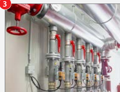
3 The heat distribution system is designed with electrically actuated valves so that each table/form/mould or bed may be heated independently from the others. Manual valves before and after the automatic valve allow for simple and quick maintenance without draining the entire system.
