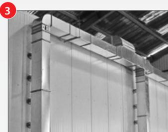
The insulated external air supply and return ducts are at the opposite sides of the curing area assuring even air flow and heat distribution. The number of distribution ducts across the length of the chamber and the number of nozzles per duct varies according to the pressure, temperature, and pallet locations in the enclosure.
