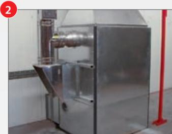
The insulated and galvanized heating unit is designed for simple connection to electrical power for the air ventilator(s), fuel source and exhaust flue for combustion.
